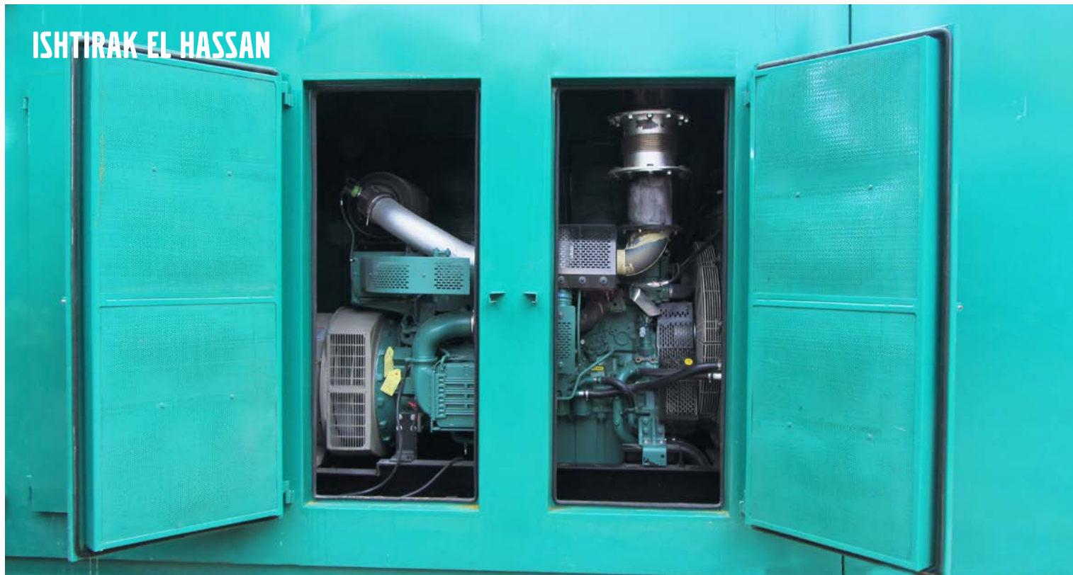
The gensets, with Volvo Penta engines, are housed in a canopy for protection against dust and rain, and for soundproofing
